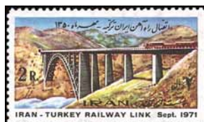
Ghatour Railroad Bridge — A364
