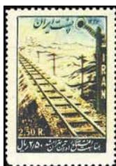
Railroad Tracks — A116
