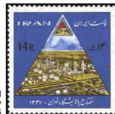
Tehran Oil Refinery A296
